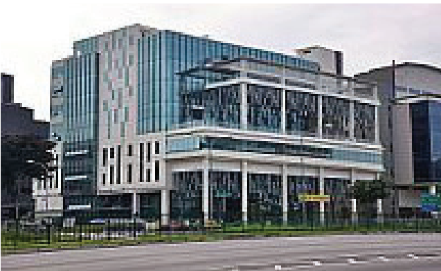
Project Title: Suki Sushi Contractor: Natural Cool Airconditioning & Engineering Pte Ltd Fan supplied: Axial, Cabinet, CIL & Propeller
