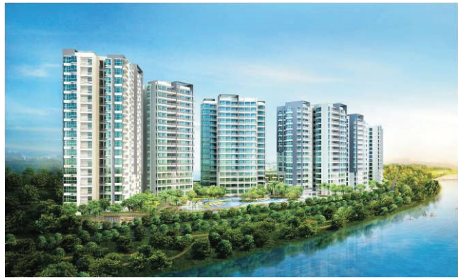
Project Title: The Estuary Contractor: Great Resources M&E Contractor Pte Ltd Fan supplied: Axial, Cabinet & CIL
